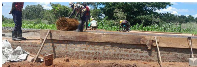
Builders laying reinforcement on the foundation wall. Cost in 2024: $7,550.88.
